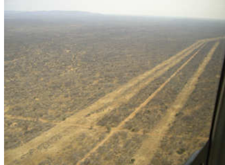
Figure 6.7 Transmission lines crossing the bushveld (seen from the air)
