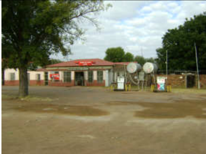
Figure 6.8 Pump station and café at Steenbokpan
