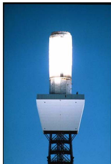
Figure 2.3: The Central Receiver - The image on the left shows the heat exchange panels, while the image on the right shows what the receiver looks like during operation (image courtesy NREL)
