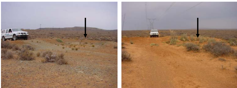
Figure 4. Examples of well constructed berms under the Hydra-Droërivier 1&3 lines. This design uses an overflow dam to spread water collected by the berm (see arrows). After ten years virtually no maintenance is required on these structures.
