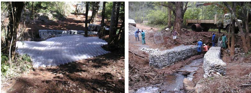
Figure 3. Extensive measures taken to prevent erosion, during the construction of access roads for a new power line. Continuous cellular mat (left) and gabions (right) are some of the measures used during the building of access roads during the construction phase of a power line. (Photos: Jose Clara).
