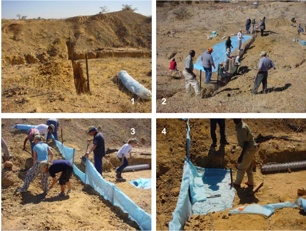
Figure 6 shows the steps in the construction of a silt-screen. Girls from two schools in Pretoria on the Mabula Game farm carried out this exercise. In photo 1 the trench is dug across the erosion channel and Y standards are placed to form the main part of the structure. In photo 2 the Y standards are connected with stay wires and covered with wire mesh. The structure is then covered with a biodegradable geo-textile in photo 3. In photo 4 the structure is completed by adding an apron, made of geo-textile and wire mesh.
