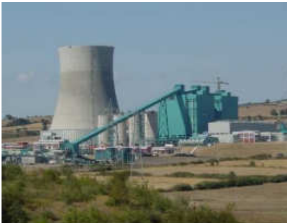
Figure 4.4 Photograph showing a power station with the dry cooling tower of the Stack-in-Tower system of indirect dry cooling technology
