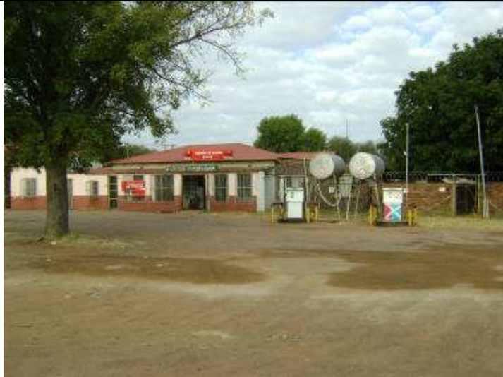
Figure 6.8 Pump station and café at Steenbokpan
