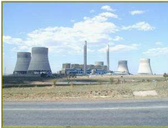
Figure 4.8 Photograph showing a power station with indirect dry cooling technology
