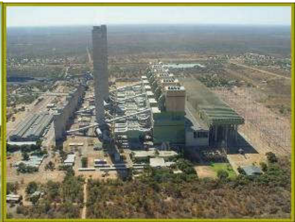
Figure 4.9 Photograph showing a power station with direct dry cooling technology
