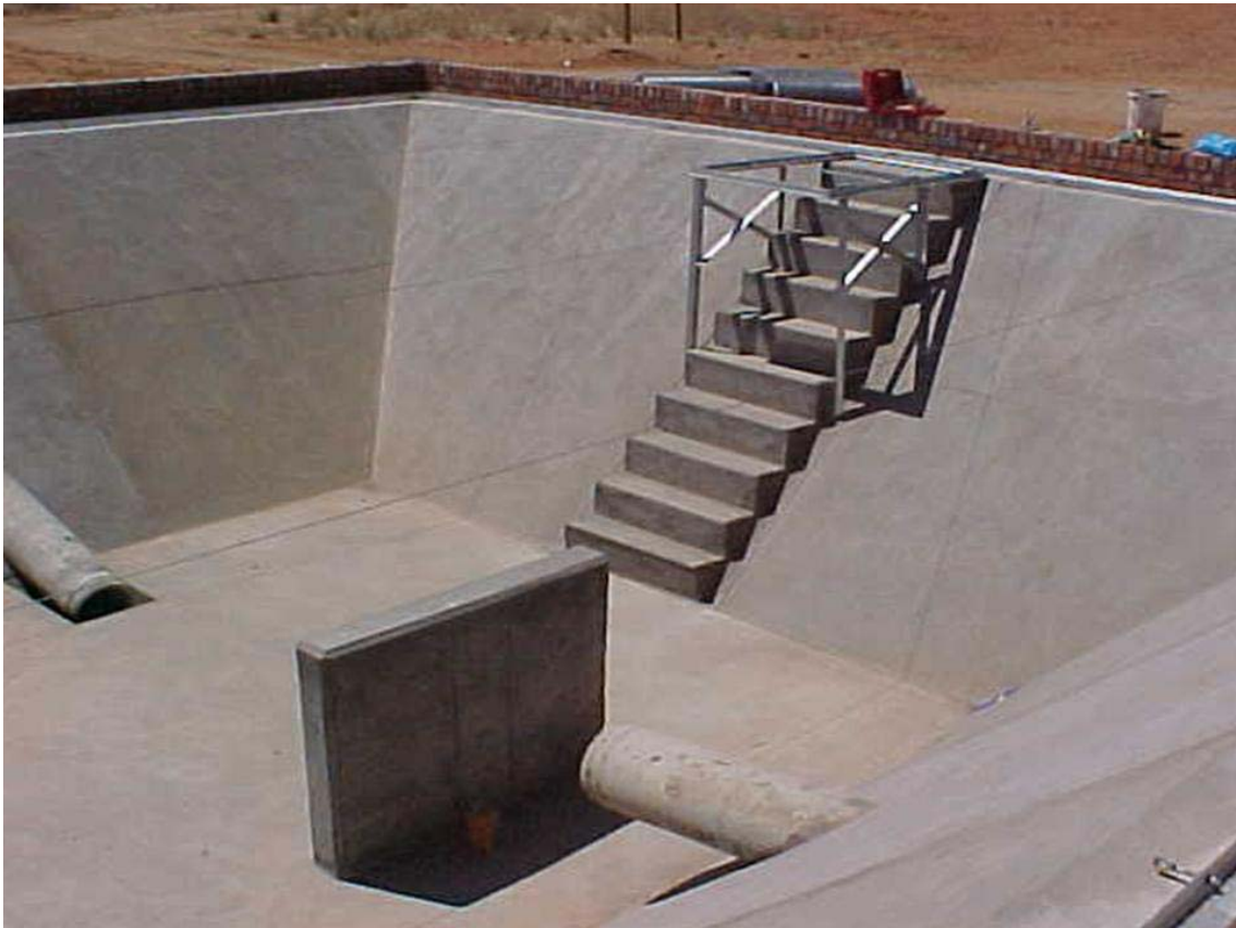
Figure 8 Oil holding dam
