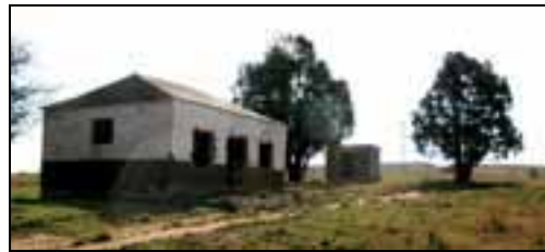
Plate 38: The building from BH14
