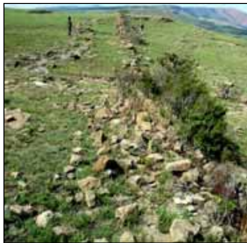
Plate 20: General view of the long stone wall
