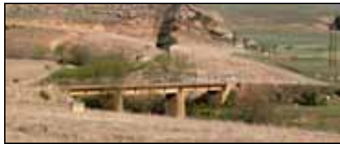
Plate 42: Bridge over the Wilge Spruit.
