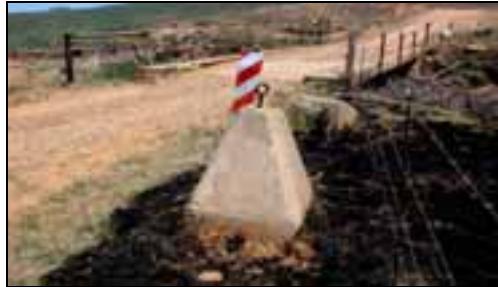
Plate 35: One of the bollards found at both ends of the bridge can be seen
