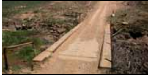
Plate 34: General view of the bridge
