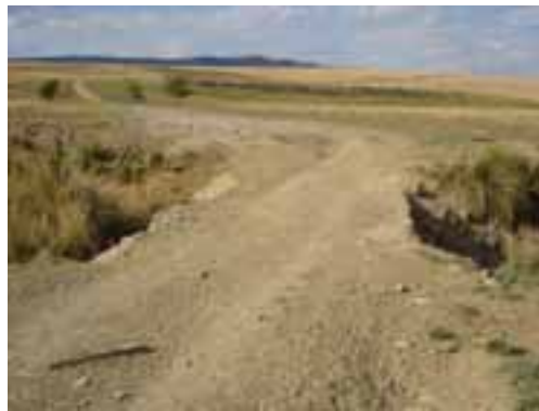
Plate 8: Inadequate storm water management structures
