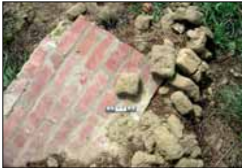
Plate 25: Remains of the farm dwelling. Note the mud bricks as well as the more conventional bricks (with cement)
