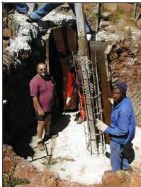
Figure 11 Pouring of concrete into a tower foundation
