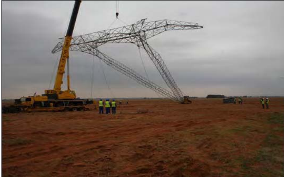
Figure 13 Illustration of a crane lifting the tower into place
