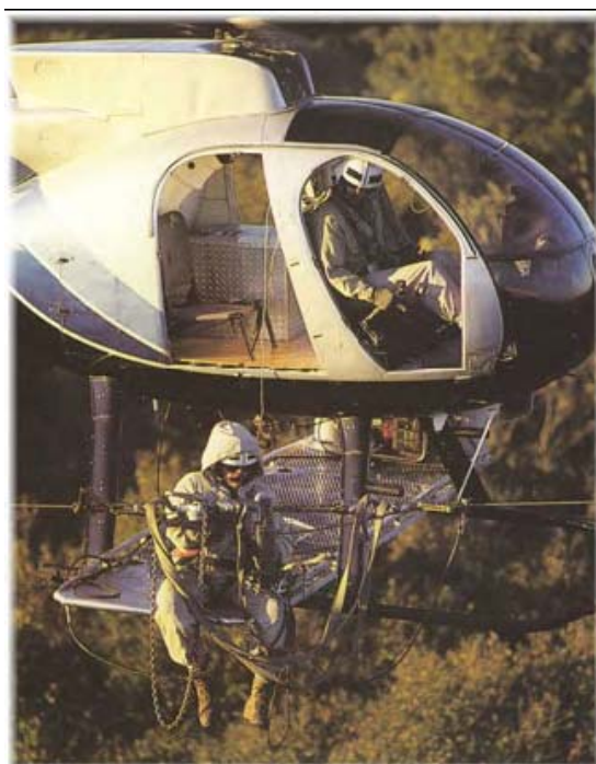
Figure 14 Maintenance undertaken by helicopter
