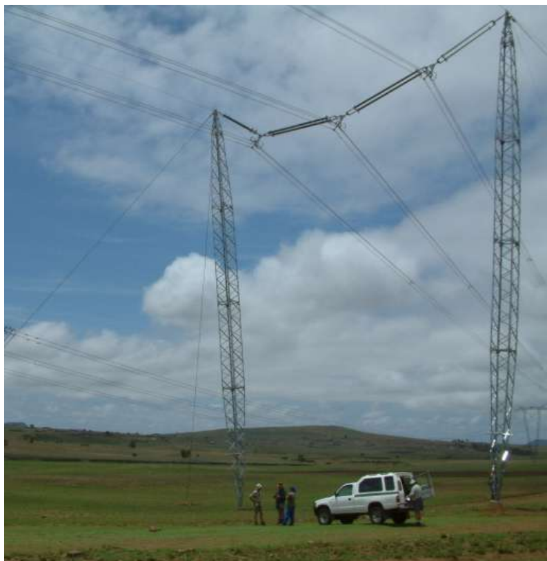
Figure 29: Cross-ropo suspension tower
