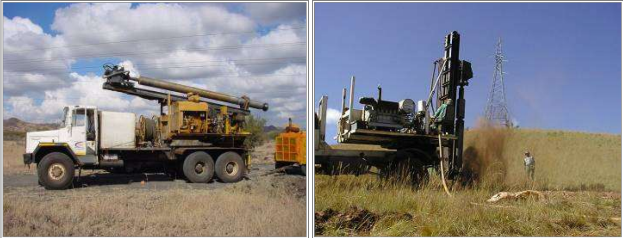
Figure 37: Drilling rig and generator (top) and excavation activities (bottom)
