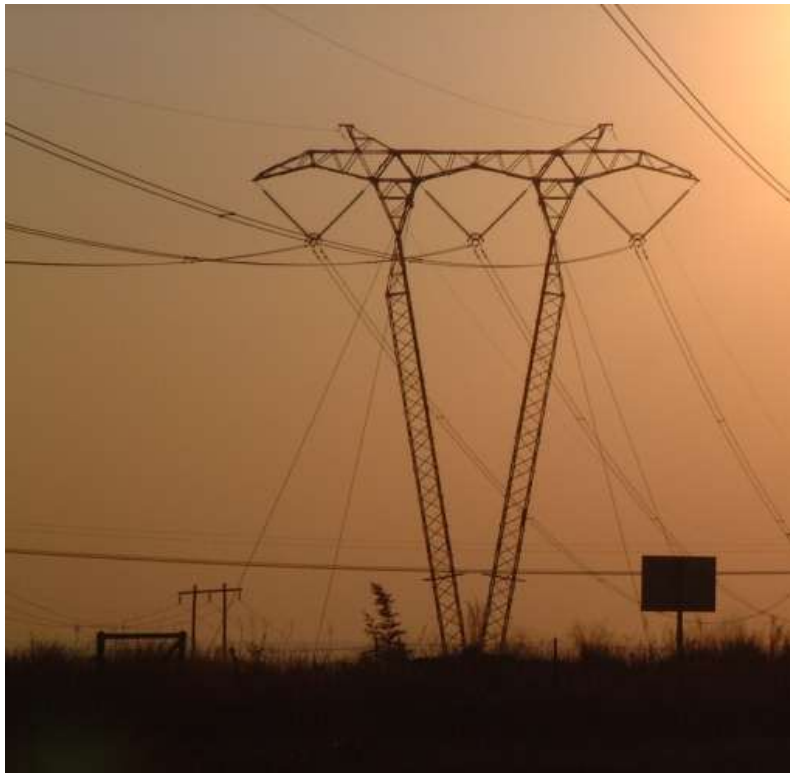
Figure 31: Guyed suspension tower
