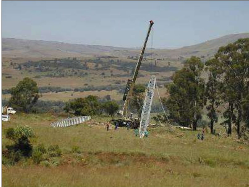
Figure 40: Erection of towers
