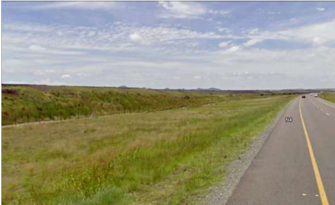
Figure 25: North-eastern view along the Western Route Alternative – Deviation 2 - route situated between the slimes dam (left) and the N4 (right)
