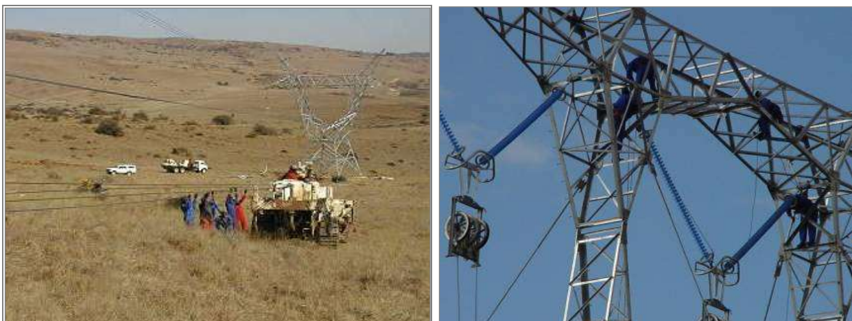
Figure 42: Stringing with pilot tractor (top) and pulleys (bottom)
