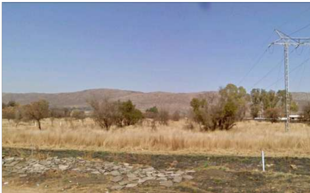
Figure 13: South-eastern view along the Eastern Route Alternative (crossing of R514, Witwatersberg in background)
