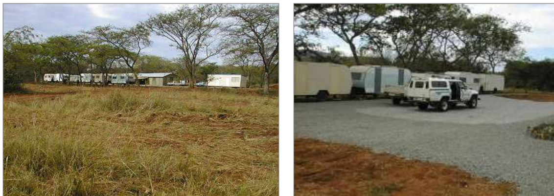
Figure 8: Examples of Construction Camps
