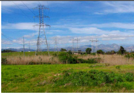
Power lines crossing wetland area, possible impact on habitat and the migration of water birds
