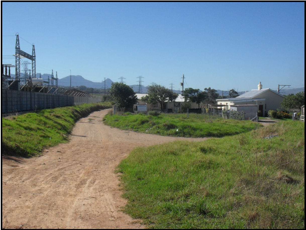
Figure 4: Houses next to the substation
