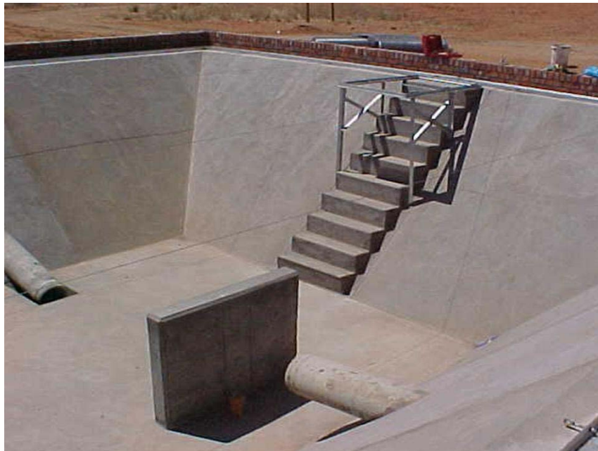
Figure 9 Oil holding dam
