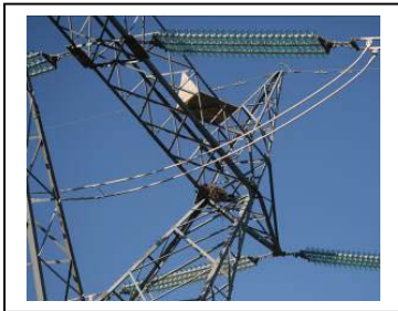
A138 Nest on 1 Droerivier Hydra Tower 178
