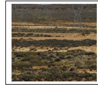
A165 Drainage line
