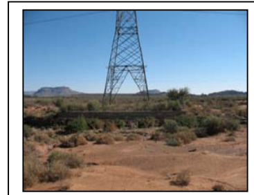
Tower A243 & B246 erosion protection near drainage line
