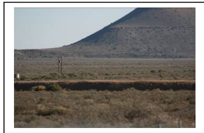
A187 – A188 & B190 – B191 Stream crossing and dam in area
