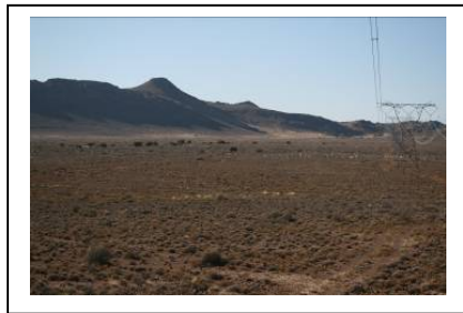
A239 – A244 Drainage line
