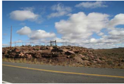
Plate 2: Shale exposed in N1 road cutting adjacent to proposed site
