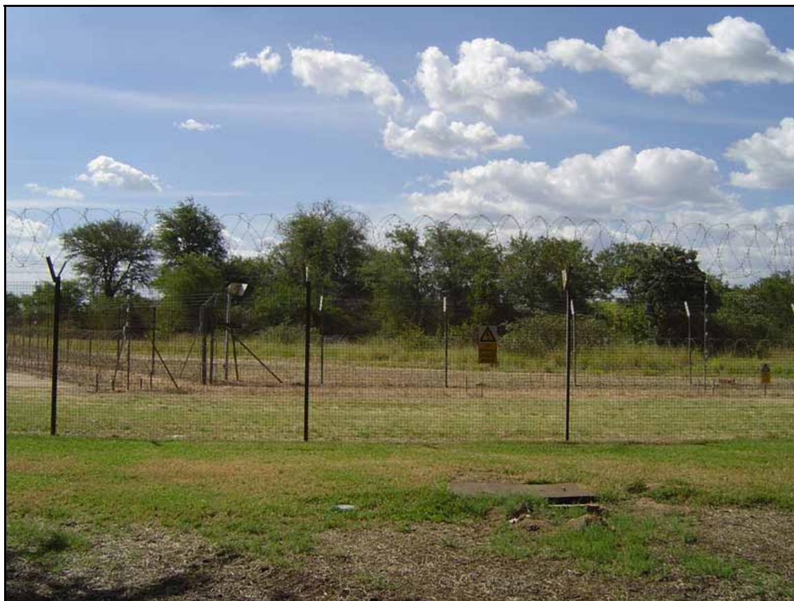
Figure 10: Matimba power station raw water reservoir security fencing. (Note: The reservoir itself is hardly visible behind the natural vegetation cover).
