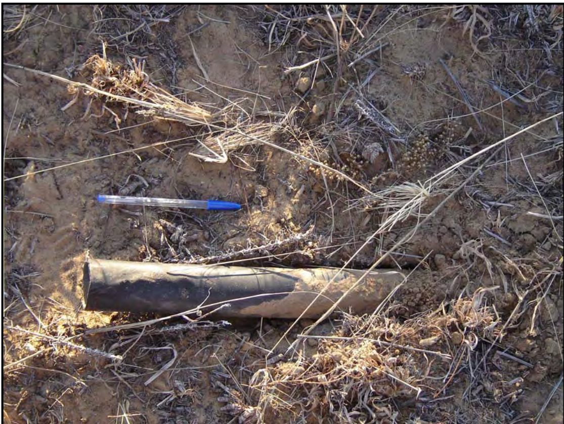
Photo 7: Buried pipe – indicating previous disturbance
