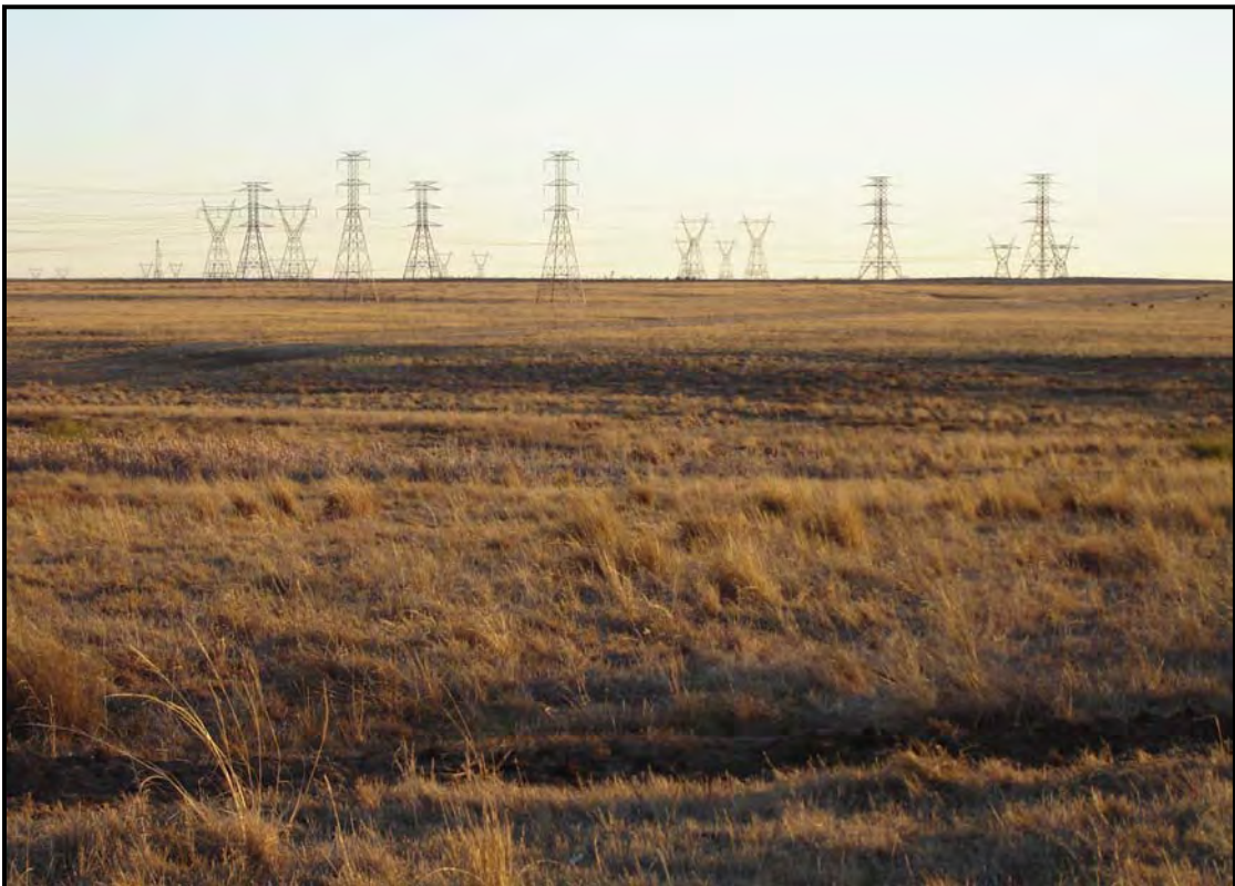
Photo 2: General view looking SE over surveyed area
