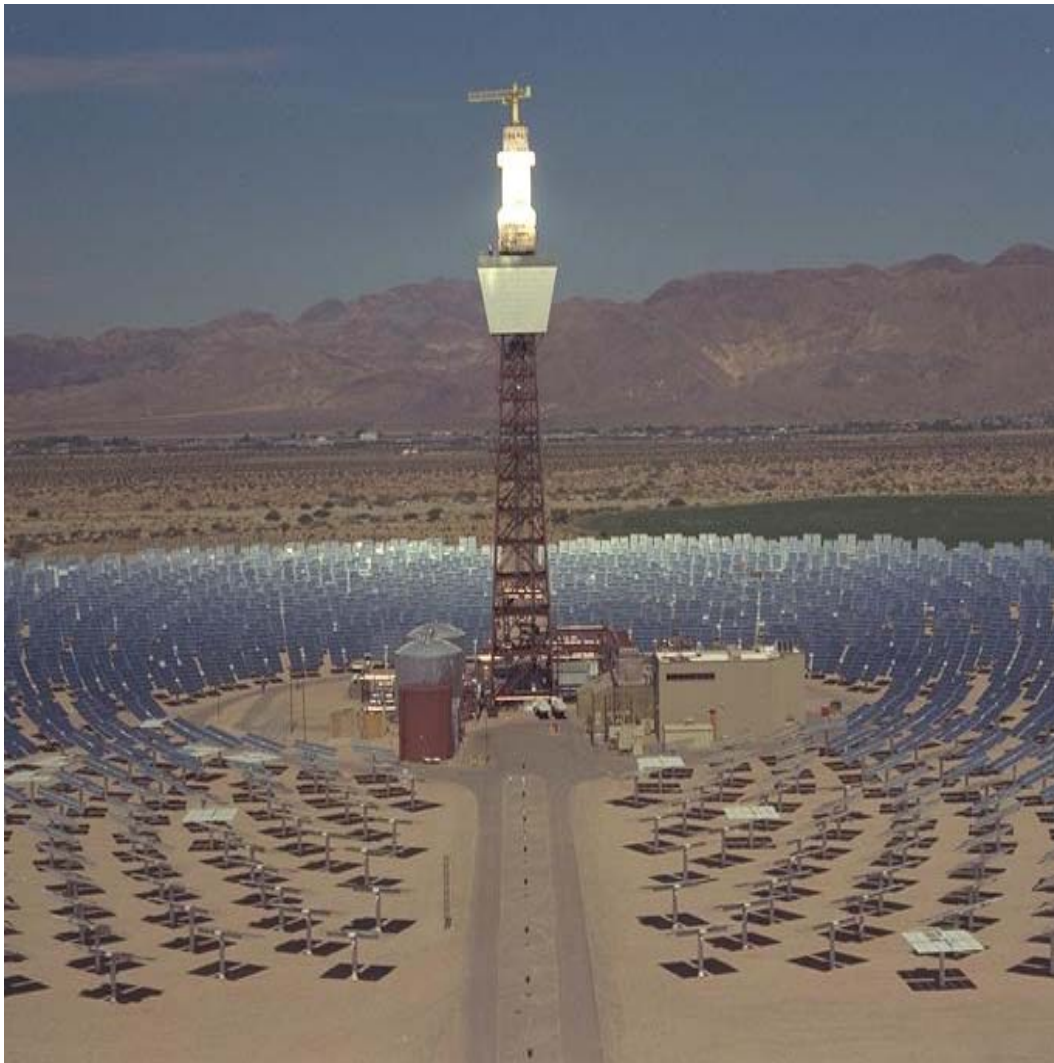
Figure 1.1: 10 MW CSP Plant constructed as a demonstration plant in the United States (Courtesy NREL).
