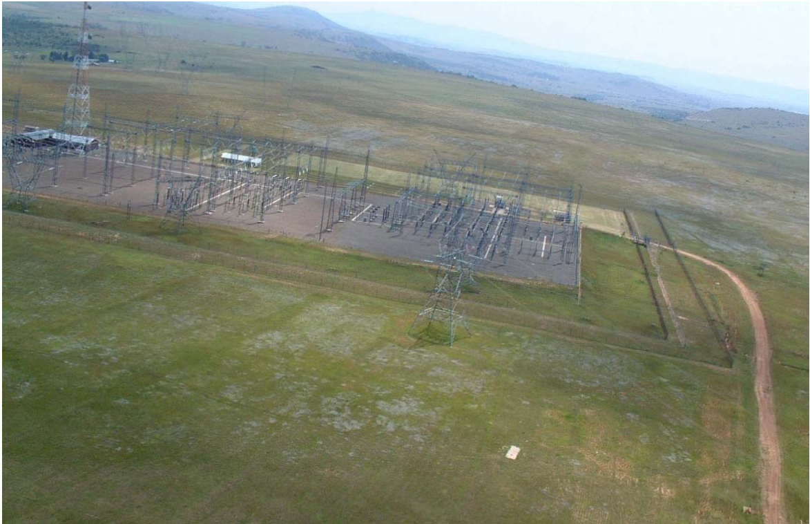
Figure 3: Example of similar substation type (Pegasus Substation, Dundee)
