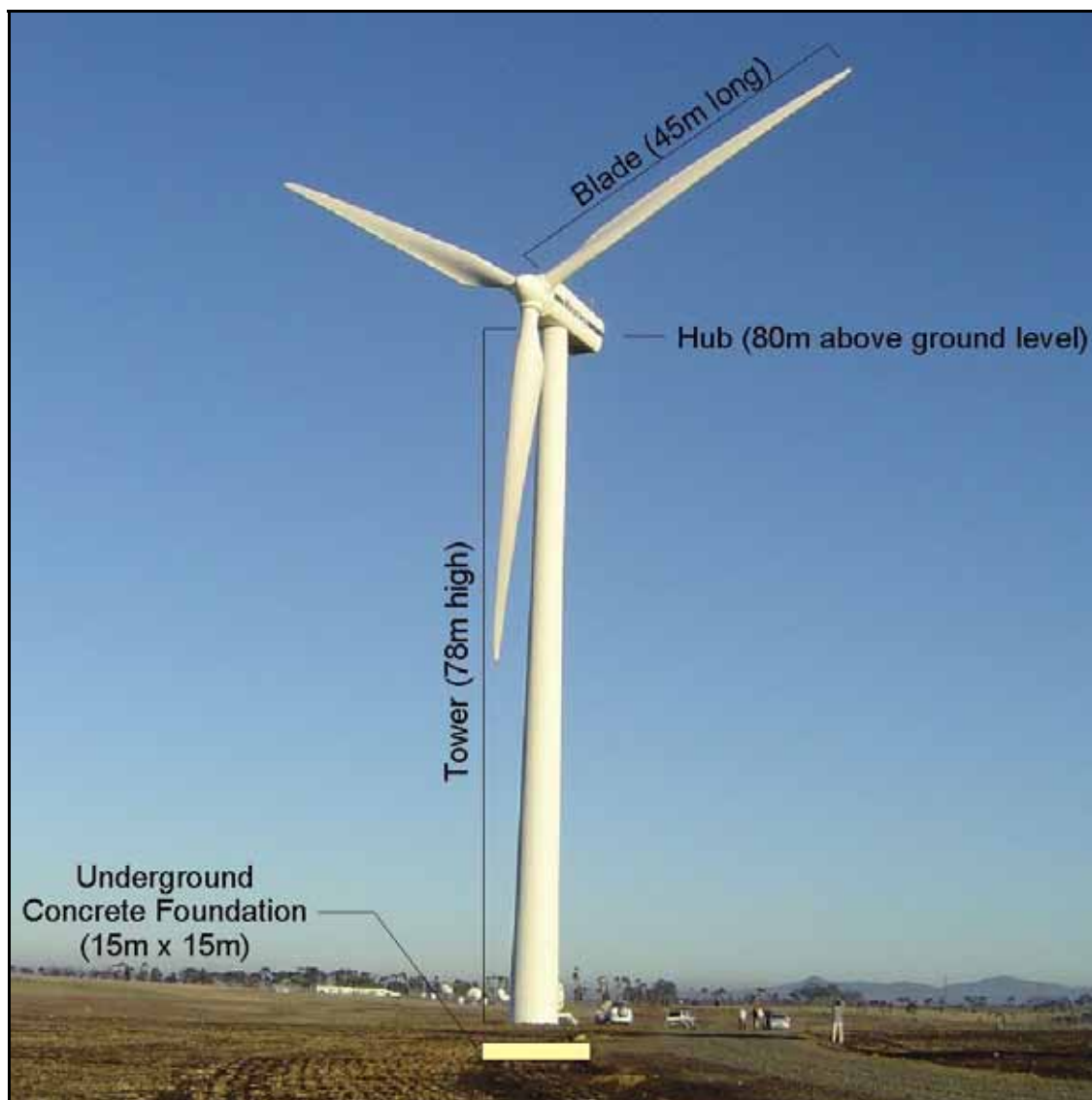
Figure 3.4: Illustration of the main components of a wind turbine (photograph of a turbine at Eskom's Klipheuwel wind demonstration facility)
