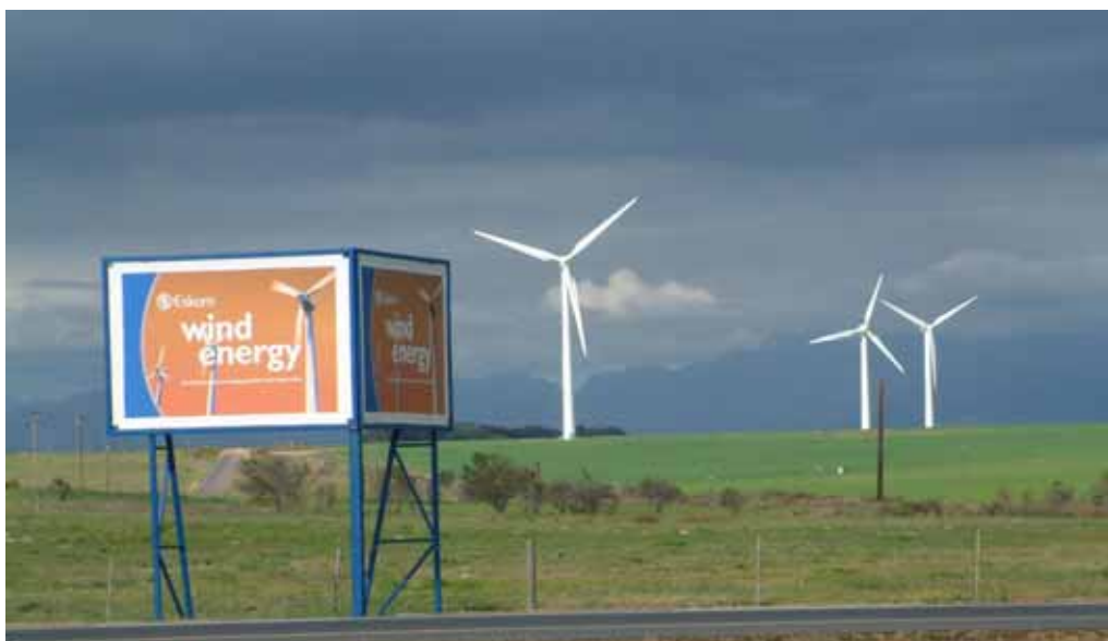
Figure 3.1: Photograph of the existing three turbines at the Klipheuvel Demonstration Facility, Durbanville
