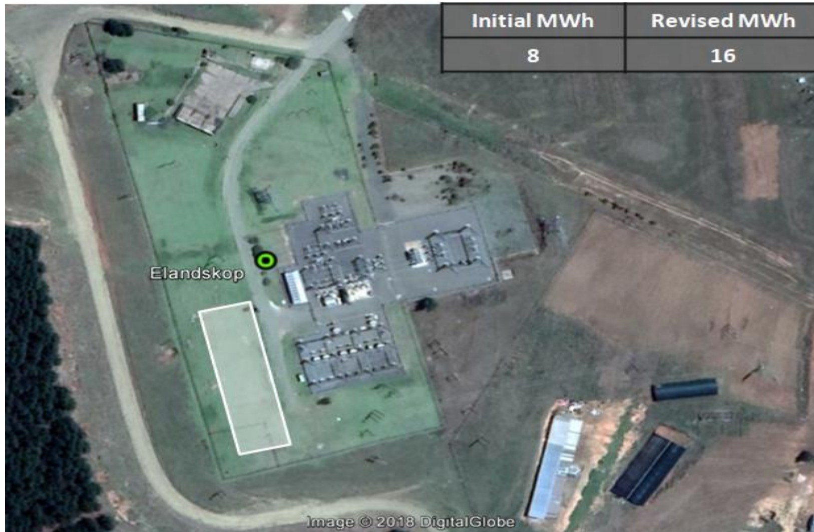
Figure 3: Elandskop Substation and Proposed Area for BESS (white), (Eskom, 2019)
