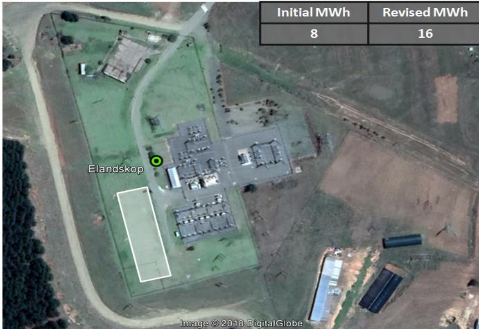
Figure 7: Location of the Proposed BESS at the Elands kop Substation
