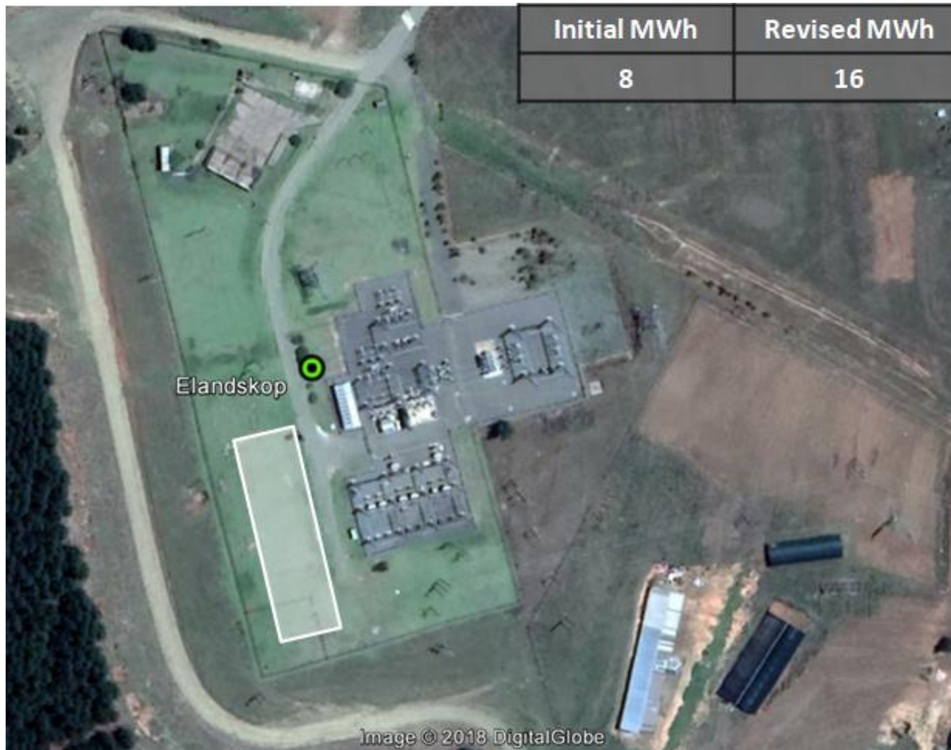
Figure 3: Elandskop Substation and Proposed Area for BESS (white), (Eskom, 2019)
