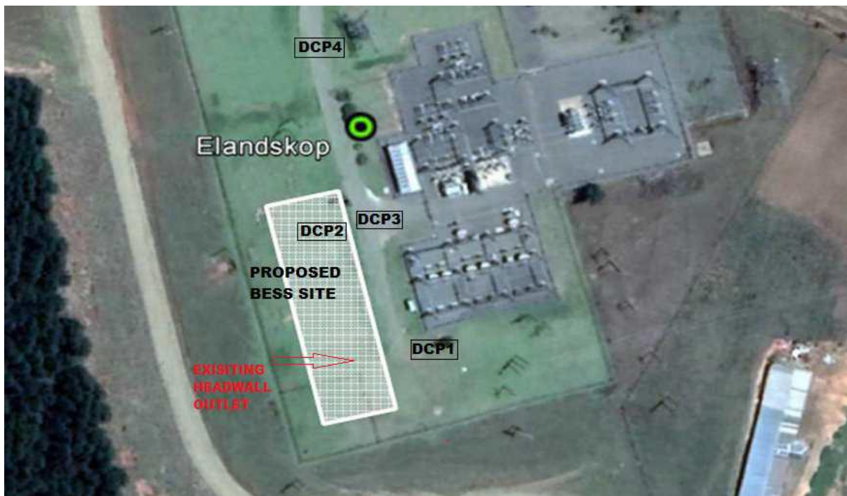
Figure 13: DCP Test Positions (Geotechnical Report, 2019)
