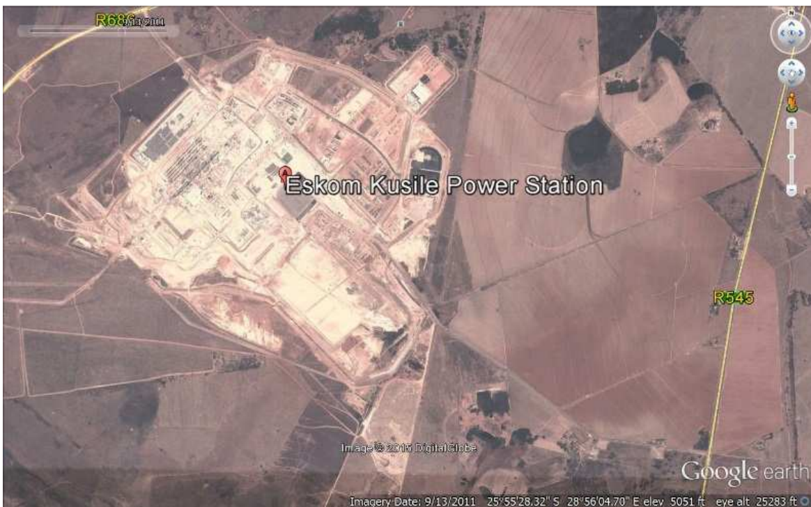
Figure 5: Google Image of Kusile Site during Construction (2011)
