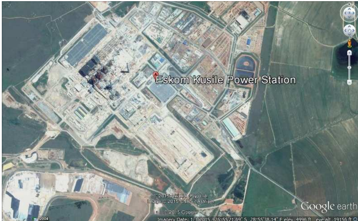
Figure 6: Google Image of Kusile Site during Construction (2015)
