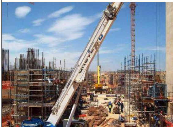
Auxiliary Bay construction - January 2010
