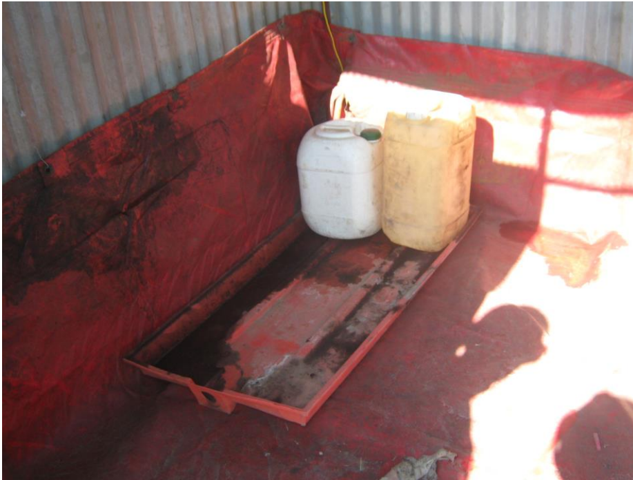
Photo 4: Plastic lining placed at the base of the hazardous storage facility.
