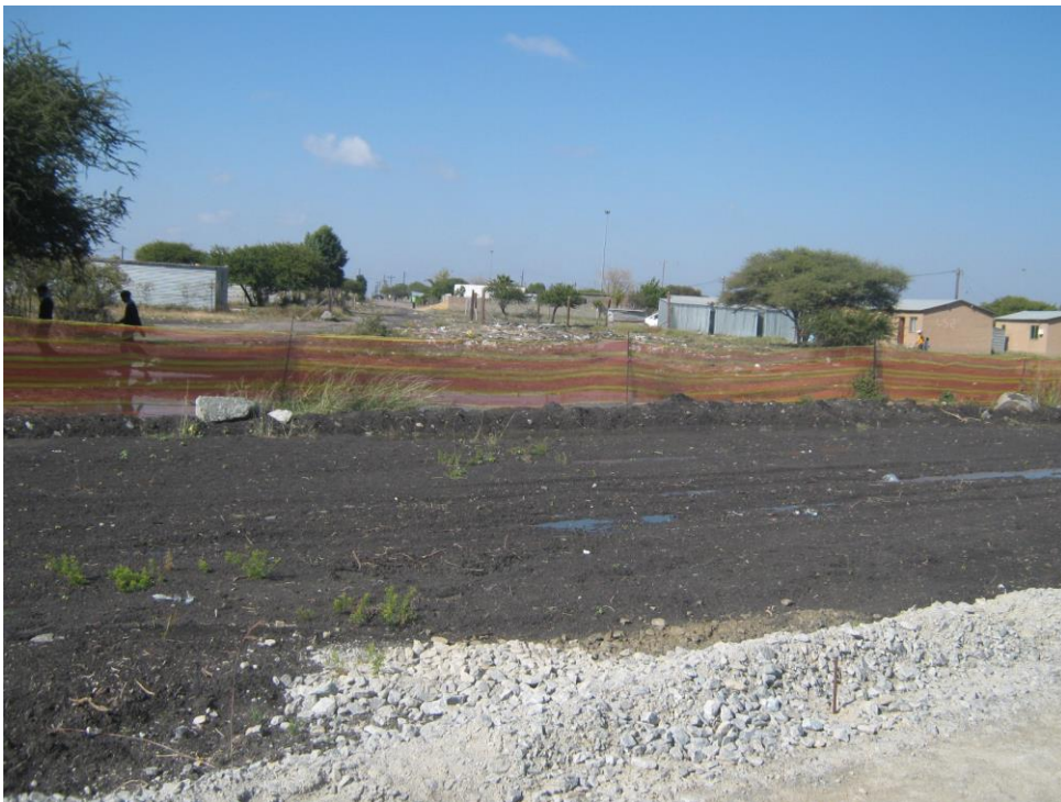
Photo 7: Evidence of weed growth on disturbed areas.
