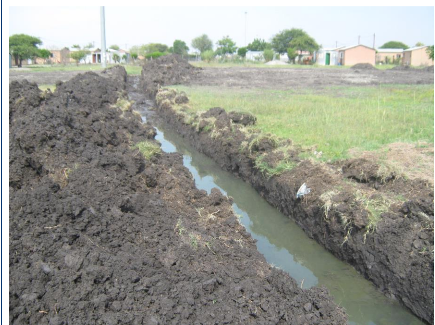
Photo 10: The cut-off trench has been upgraded.
