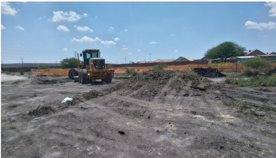
Photo 4: Topsoil stockpile stacked away
