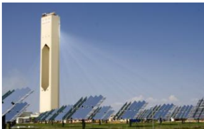
Figure 2: CSP in Seville, Andalusia, Spain.
