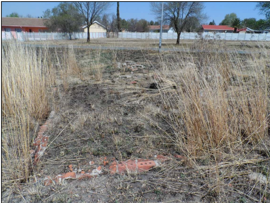
Figure 13 - Red clay brick foundations
