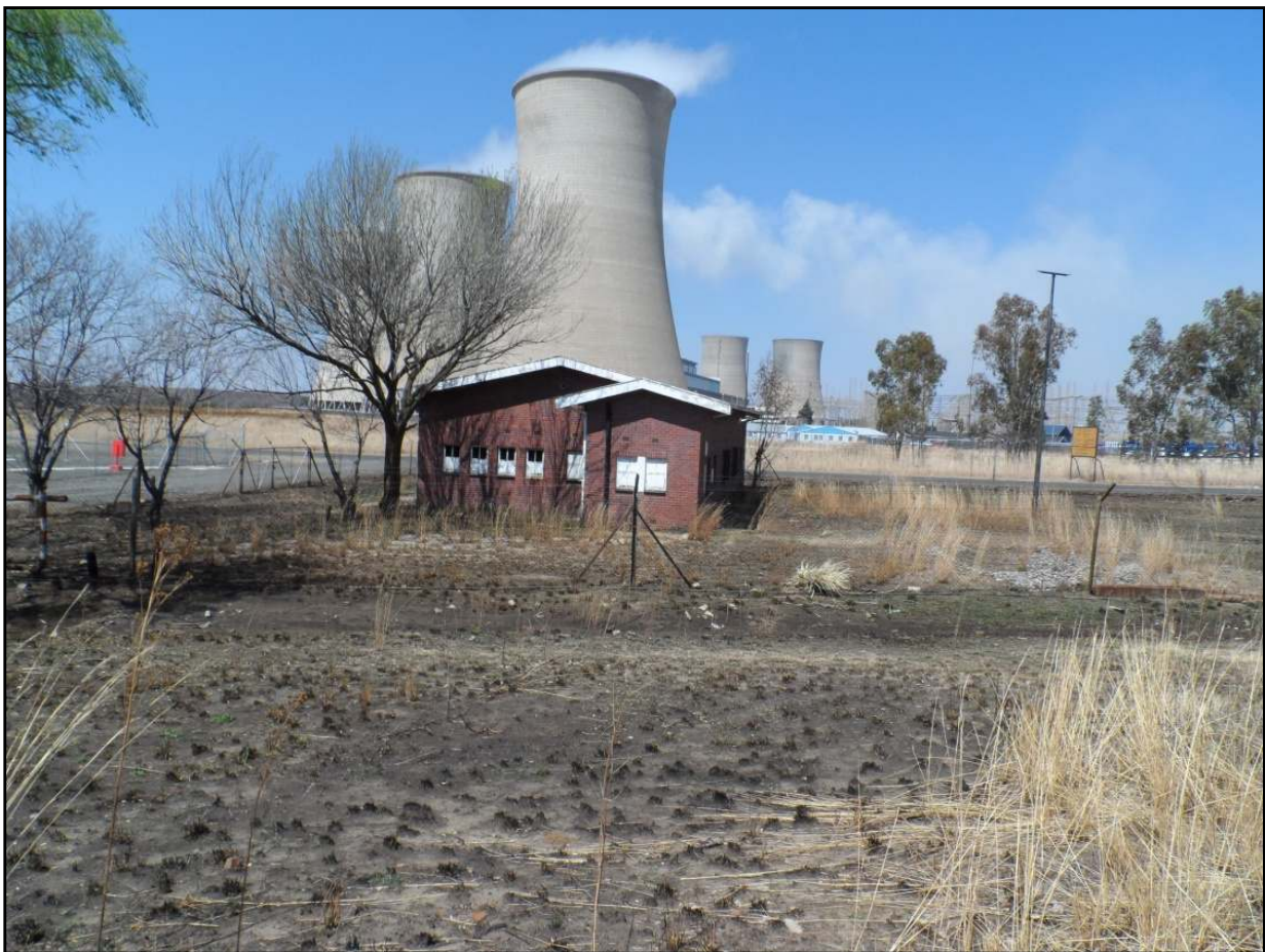
Figure 15 – Red clay brick structure located in close proximity to Eskom Plant and cooling towers.
