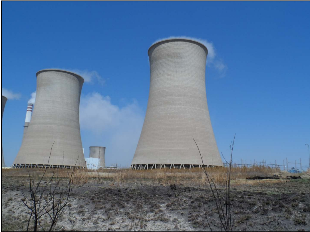
Figure 4- Eskom cooling towers in area 4
