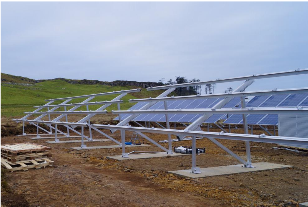
Figure 6: Typical ballast foundations
