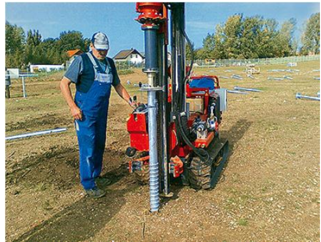
Figure 2: Typical machine used to screw the piles into the ground
