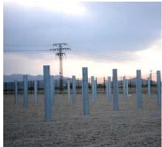
Figure 4: Rammed piles
