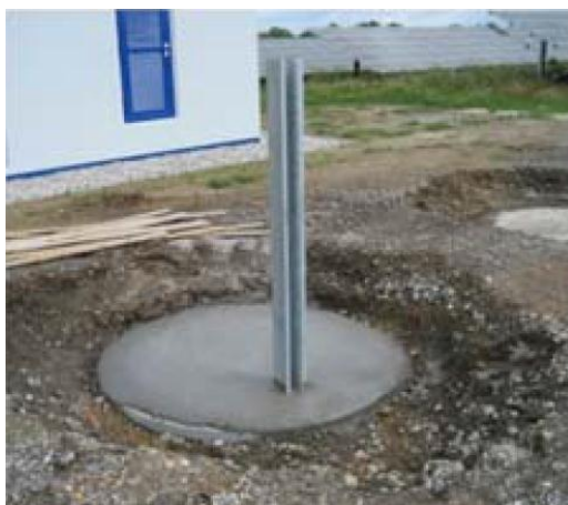
Figure 5: Typical concrete filled foundation
