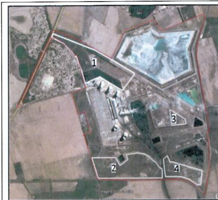
Figure 1: The original sites identified for placement of the proposed PV facility around the power station – Alternative 4 is being considered further in the BA process
