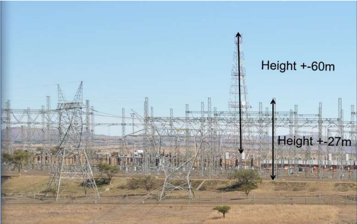
Figure 3.2: Side view of typical substation site
