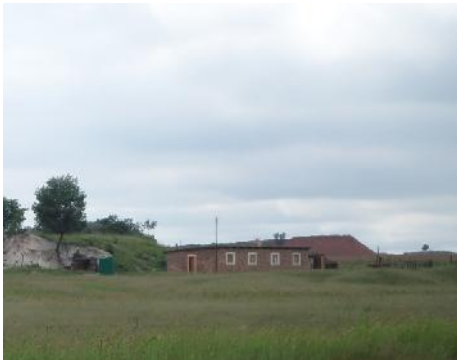
Figure 9: Houses east of the R545 (near Kendal Power Station)
