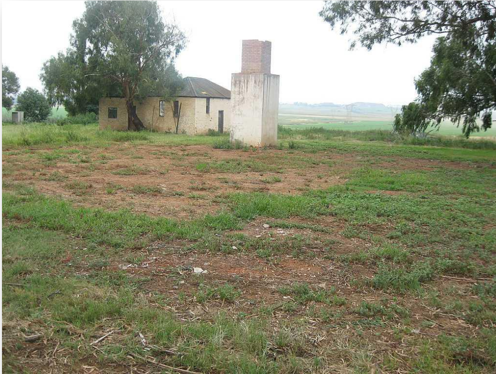
Figure 23 – Water tower at the back of building
