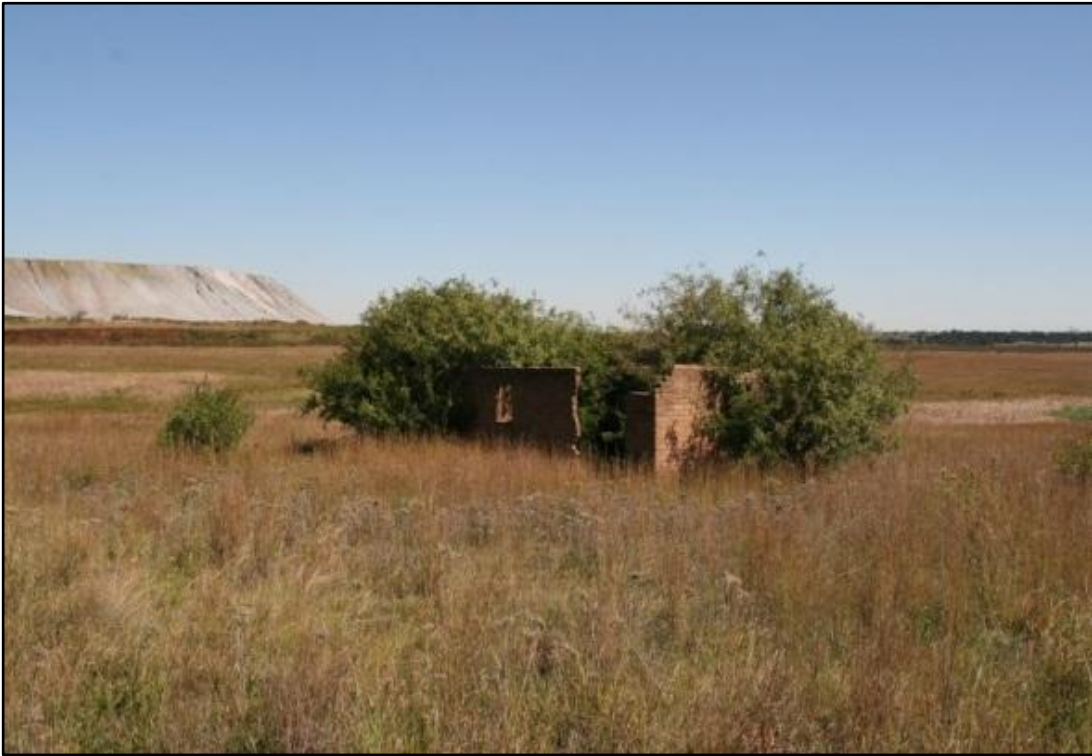
Figure 7-8: Structure as viewed from the east towards the existing ADF 34
