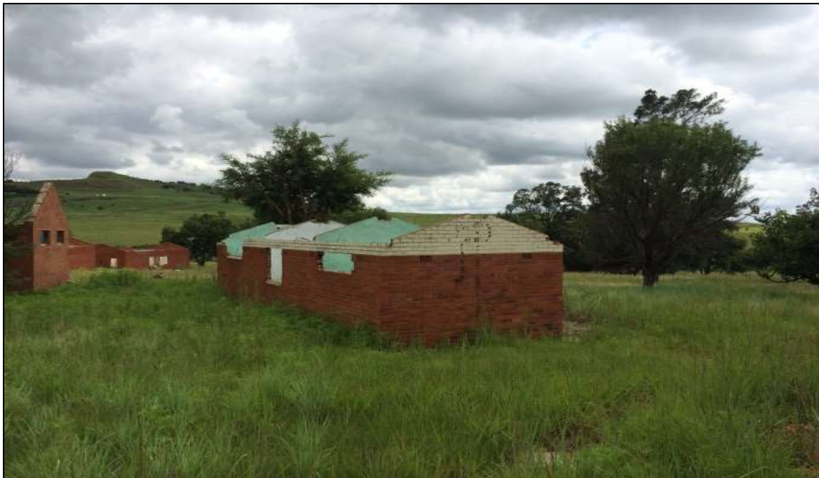
Figure 5-5: Remnant infrastructure north of the Discard Dump
