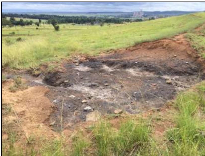
Figure 5-3: Sheet erosion and underlying discard material on the Discard Dump
