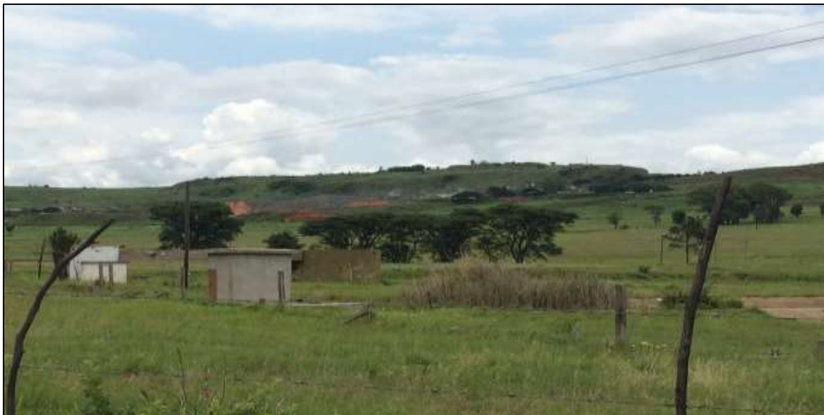
Figure 5-6: Decommissioned WWTP north of the Discard Dump
