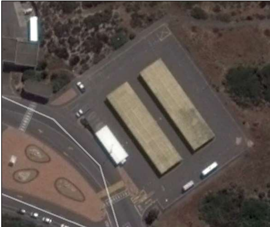
Figure 12: Aerial view of the Transport Garage site (Alternative 2).
