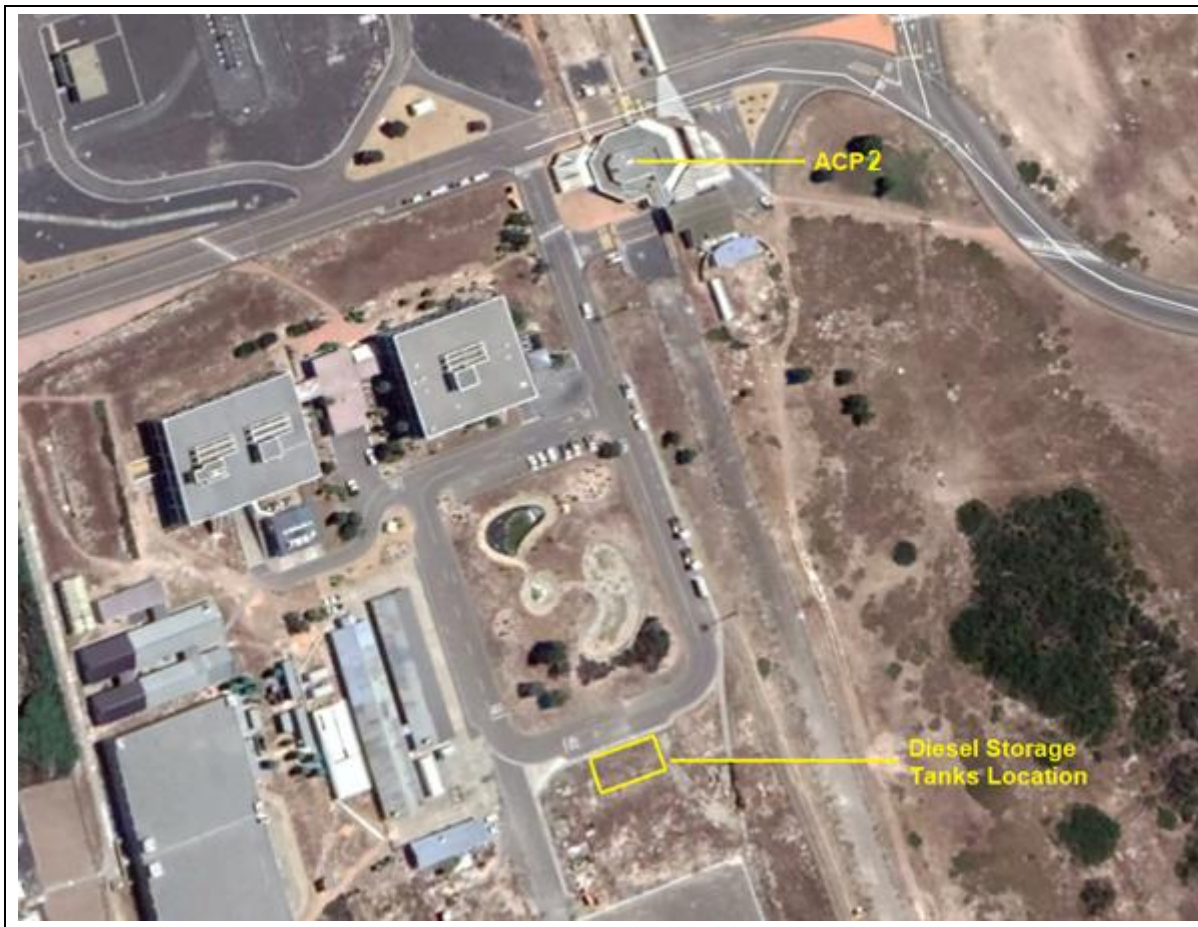
Figure 1: Site Location at the Koeberg Nuclear Power Station (KNPS)
