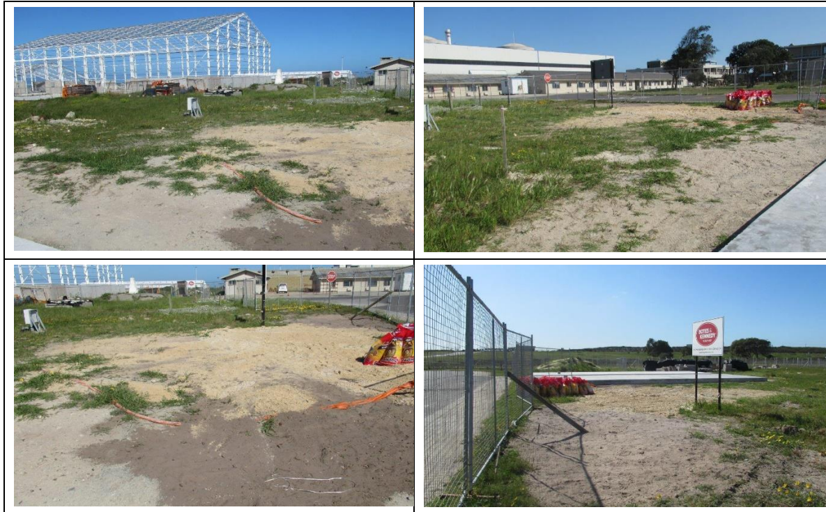
Figure 4: Close out site inspection
