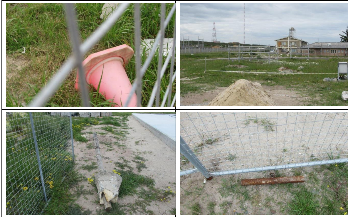
Figure 3: Pre-close out site inspection
