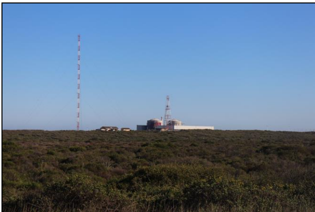
Figure 3: KNPS as viewed from the Duynefontein residential area
