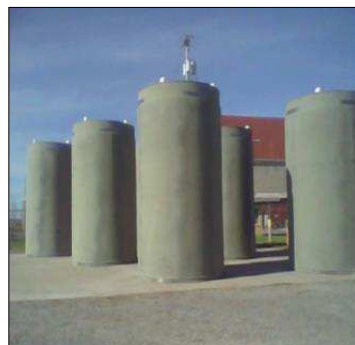
Concrete dry storage casks
