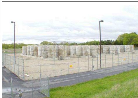
TISF comprising a concrete slab onto which dry storage casks can be placed, with a secure perimeter fence
