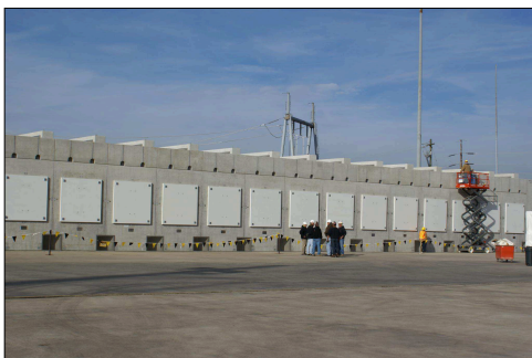
Horizontal concrete systems
