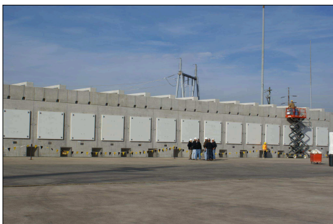
Horizontal concrete systems
