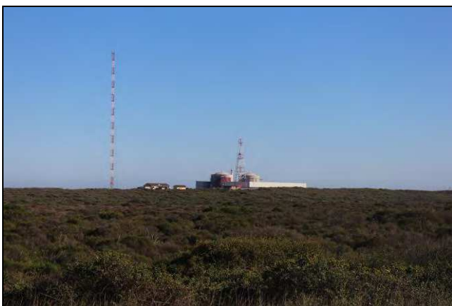
Figure 3: The KNPS as viewed from the Duynfontein residential area
