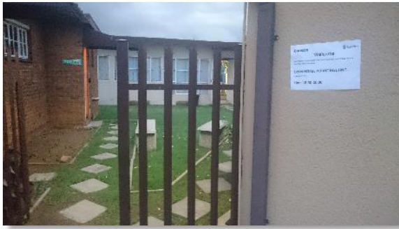
Figure 14 | Entrance to the Kriel Methodist Church
