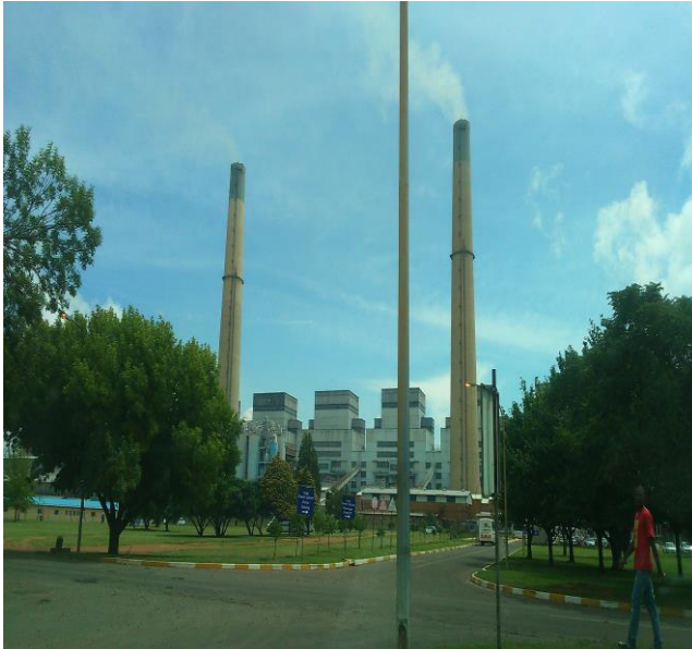
Figure 4: Kriel Power Station
