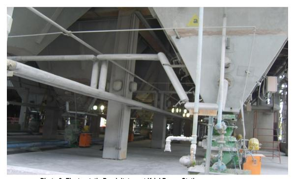
Photo 2: Electrostatic Precipitators at Kriel Power Station
