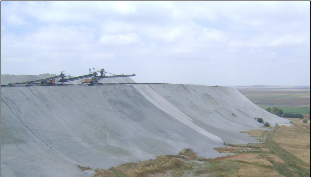
Figure 9-2: Typical stacking ash at angle of repose (as seen at Kendal Power Station)
