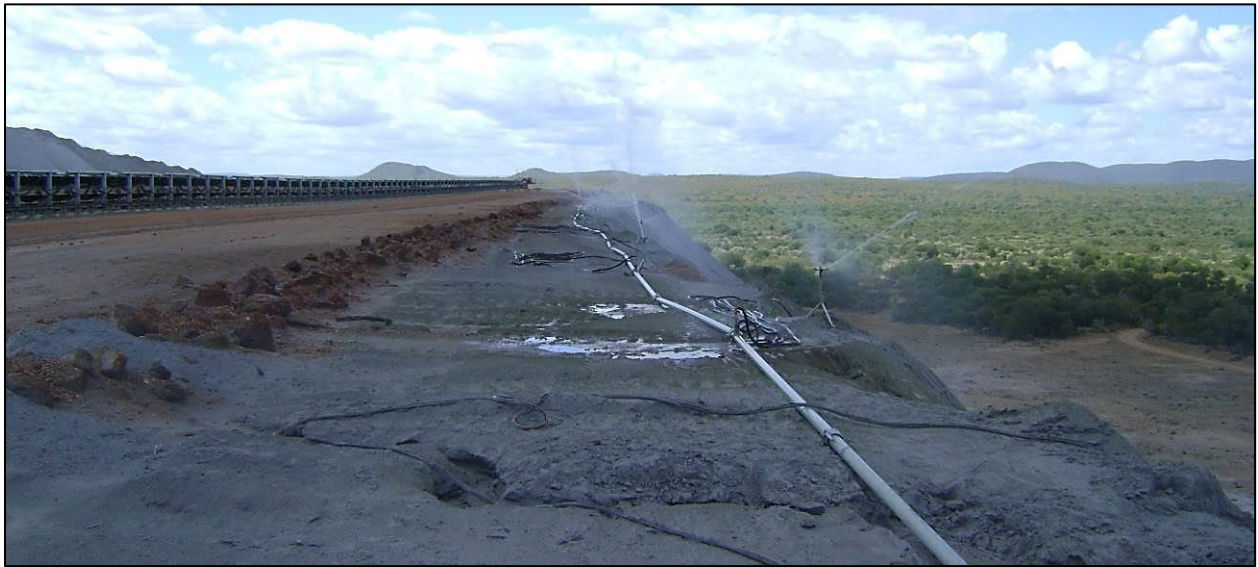
Figure 8-11: Dust suppression system at Matimba Power Station
