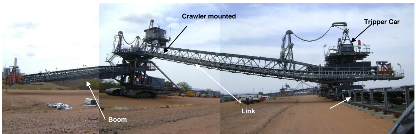
Figure 8-8: Stacker setup at Medupi Power Station
