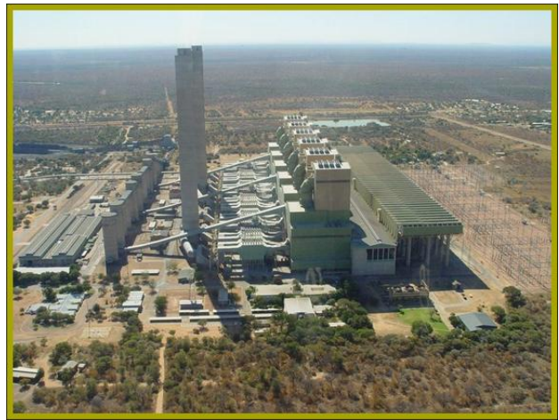
Photo 2.2 Direct dry-cooled power station
