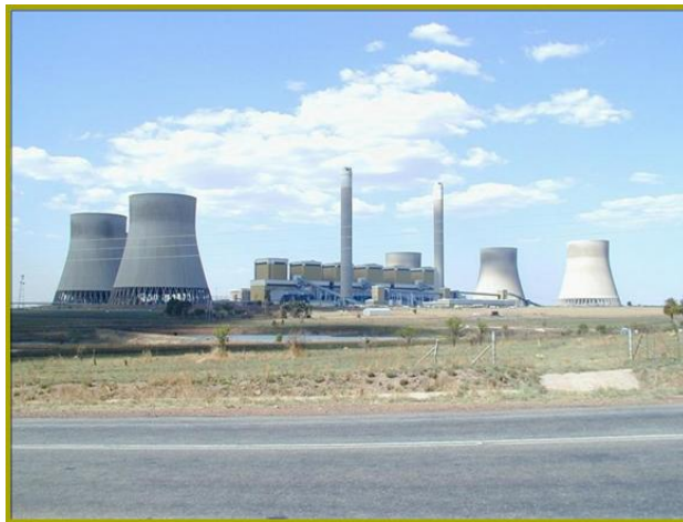
Photo 2.1 Indirect dry cooled power station
