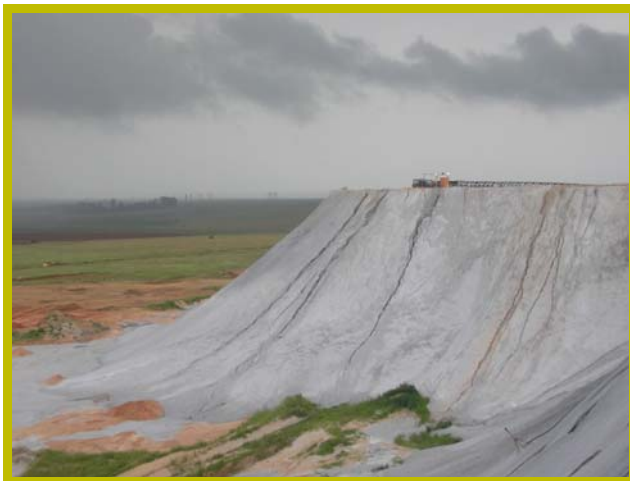
Photo 4 Above-ground ash dump
