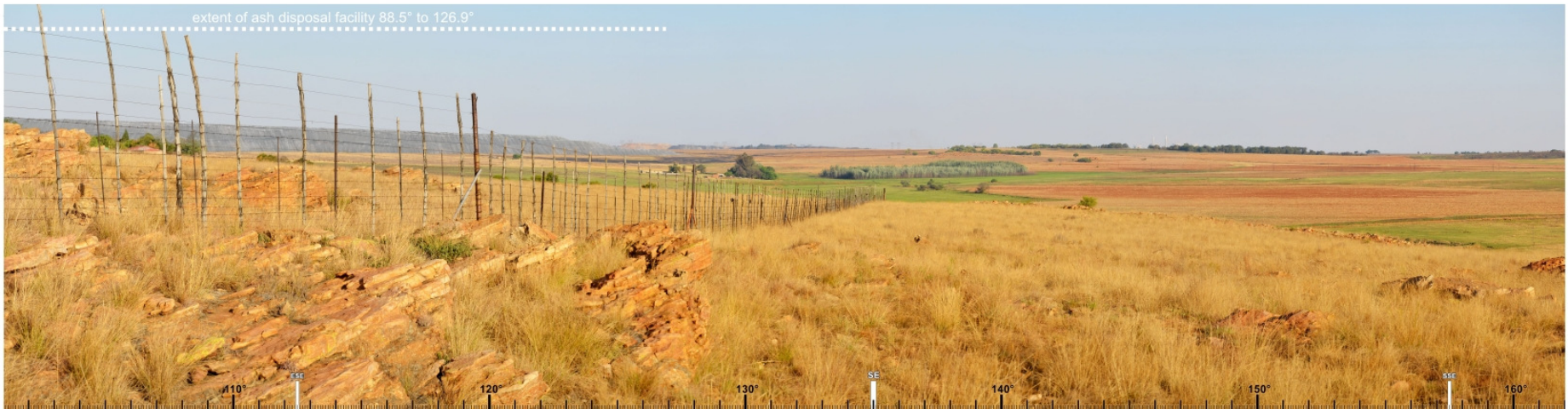
simulated view of proposed ash disposal facility at the end of its life time (60 years) and with no mitigation measures applied, i.e. worst case scenario
