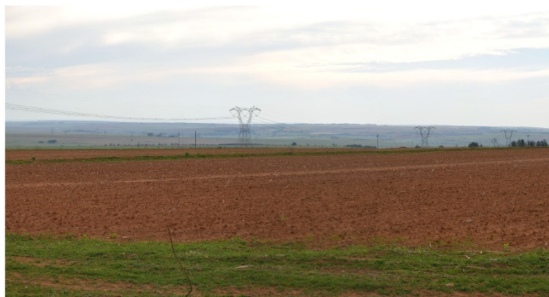
View 15: power lines
