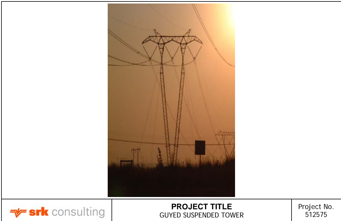
Figure 4-7: Guyed suspension tower
