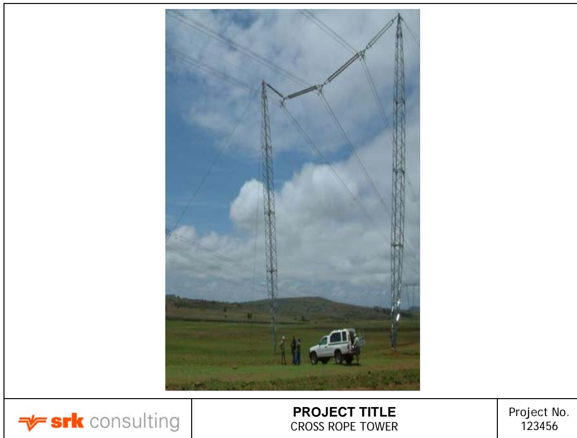
Figure 4-8: Cross rope tower
