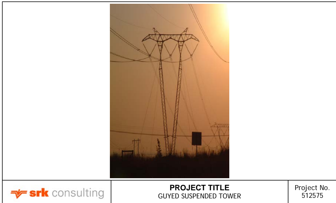
Figure 4-7: Guyed suspension tower
