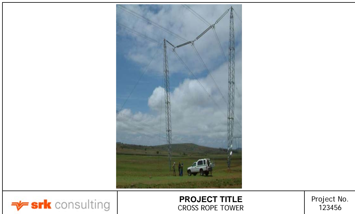
Figure 4-8: Cross rope tower
