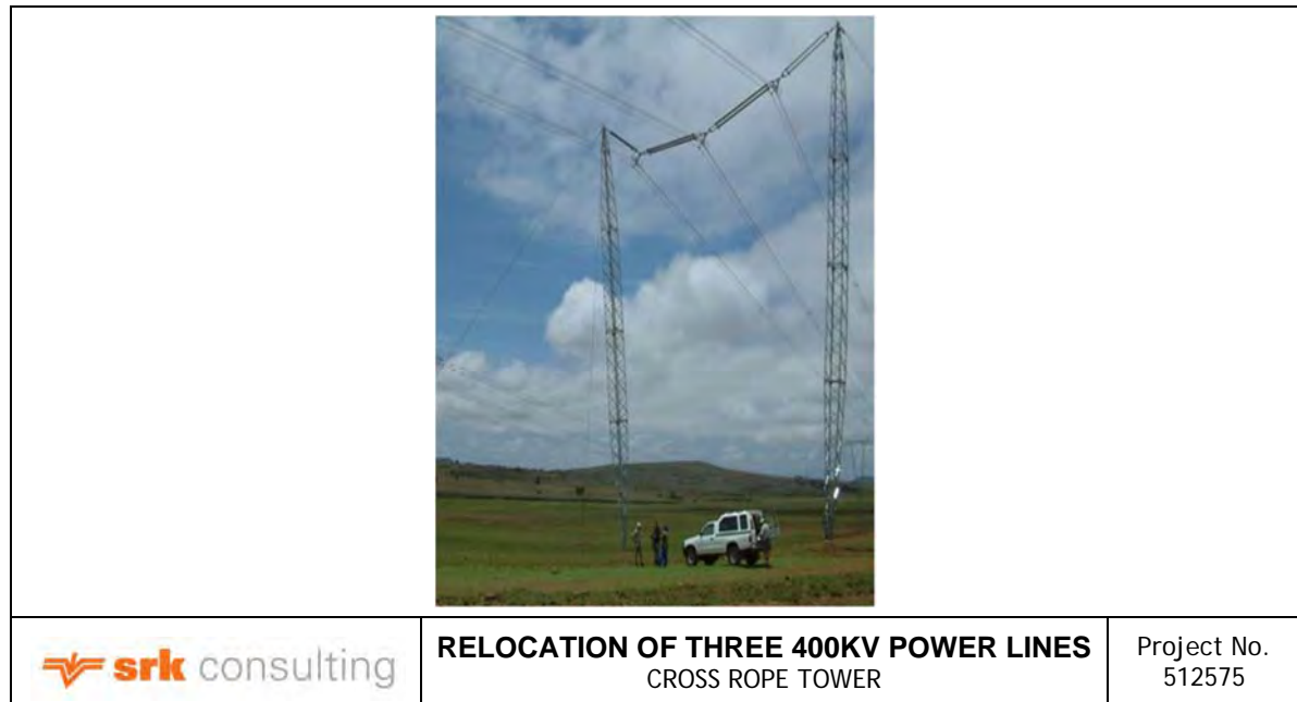
Figure 4-8: Cross rope tower
