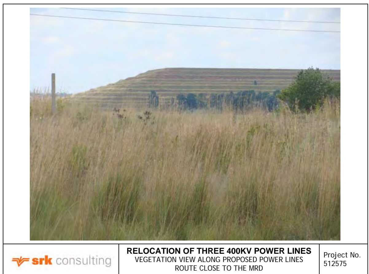
Figure 5-43: View of vegetation along the proposed power lines route close to the MRD
