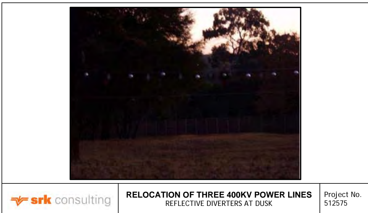
Figure 5-20: Reflective diverters at dusk with conventional white bird flappers in between (Van Rooyen, 2009)
