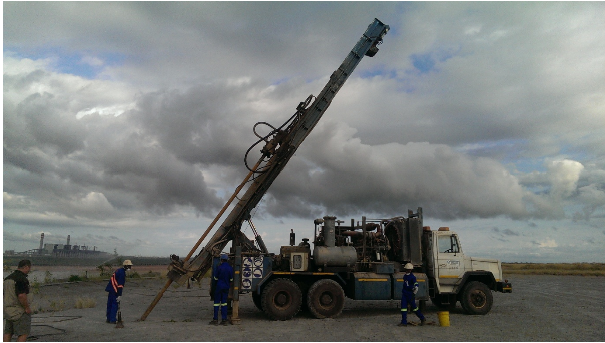
Figure 2 - Establishing Borehole
