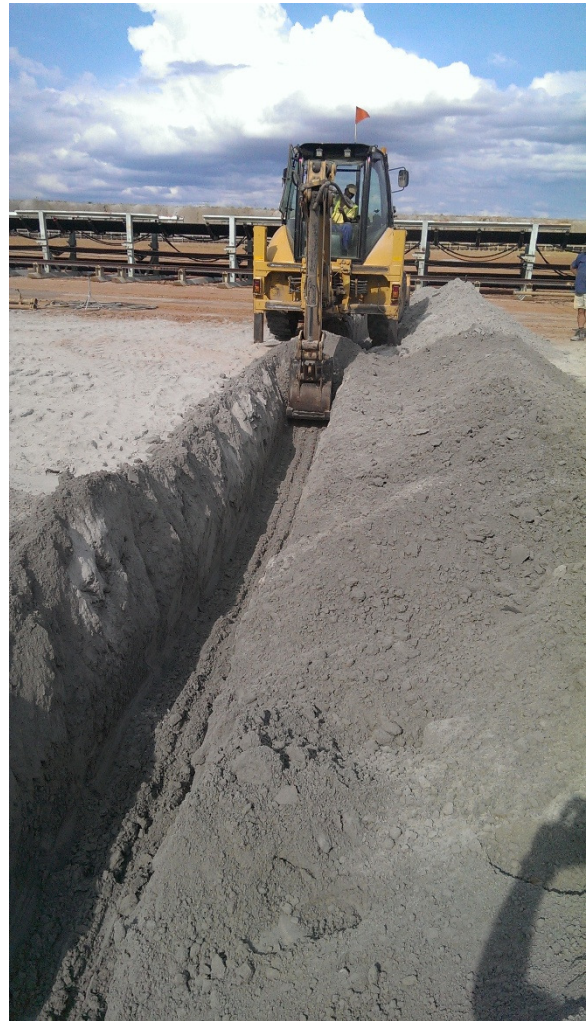
Figure 7 - Excavation of Trench to Establish Thermal Test Station 4
