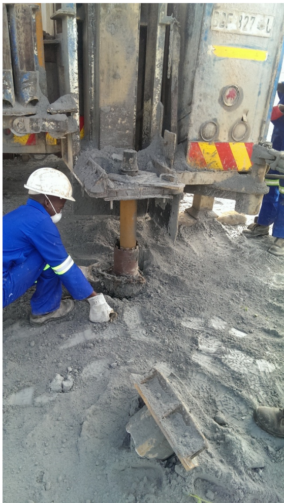
Figure 4 - Sinking Borehole Shaft
