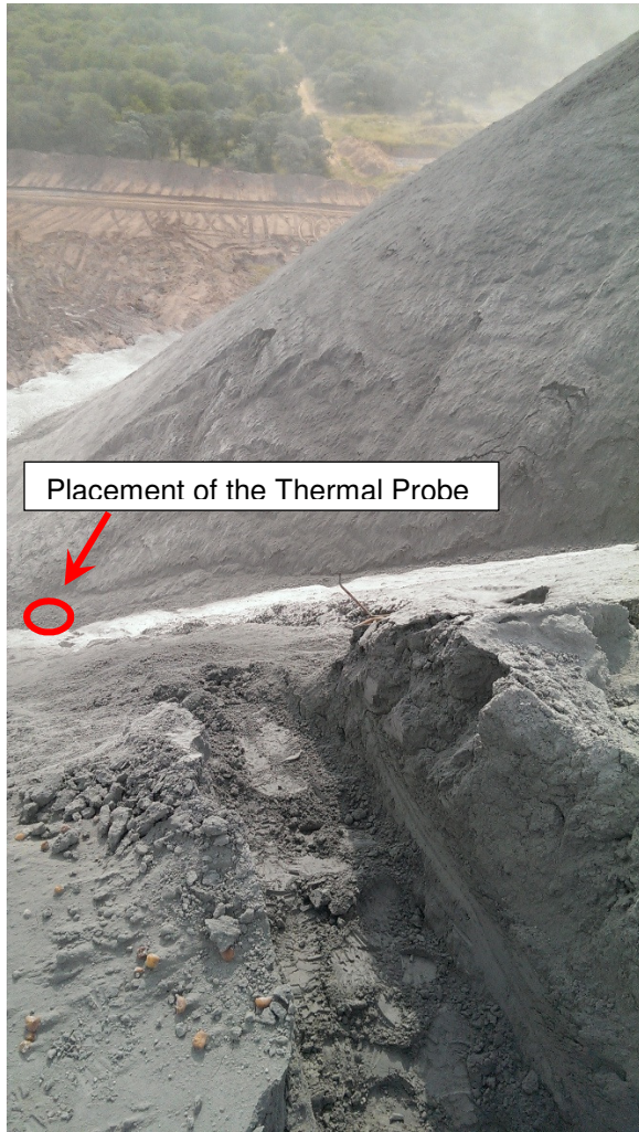
Figure 8 - Placement of Thermal Probes into Advancing Ash Pile
