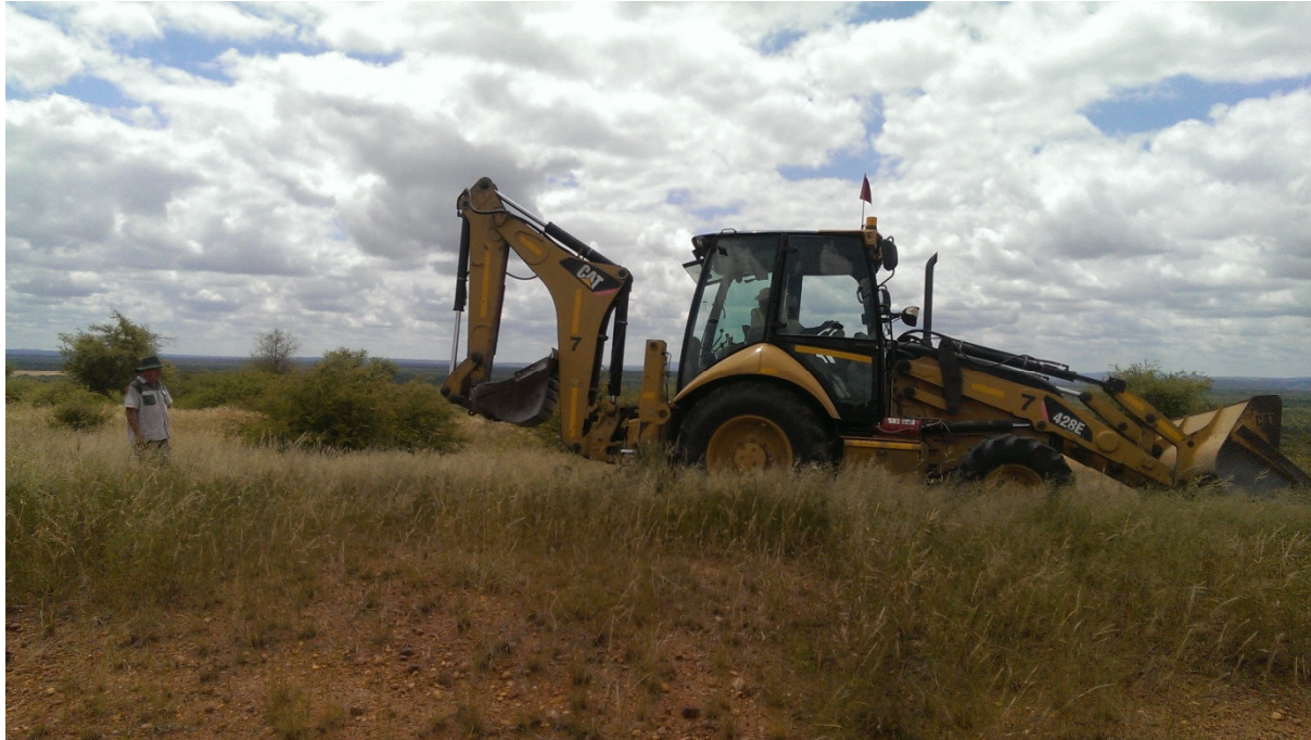
Figure 18 - TLB and engineer enroute to a trial pit on-site
